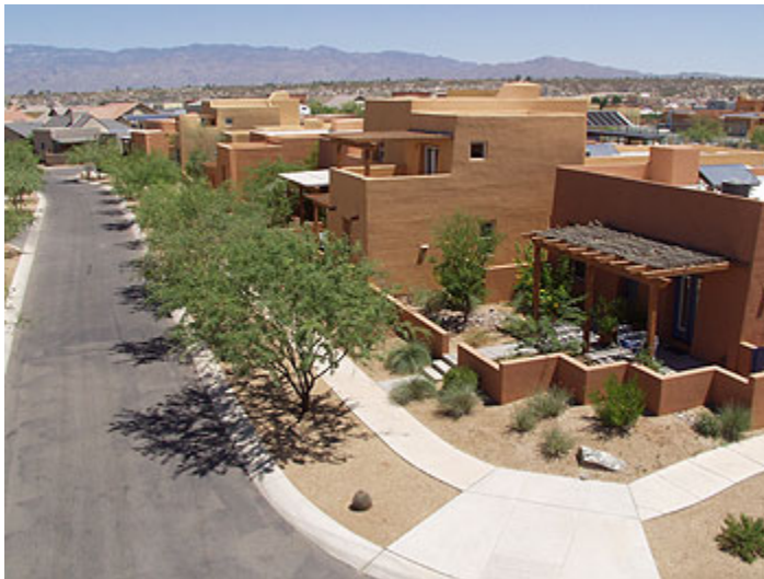
While solar hot water heating is standard on most homes in the Tucson, Arizona, community of Civano, many homes also feature solar photovoltaic panels. Photo courtesy Community of Civano, LLC.
