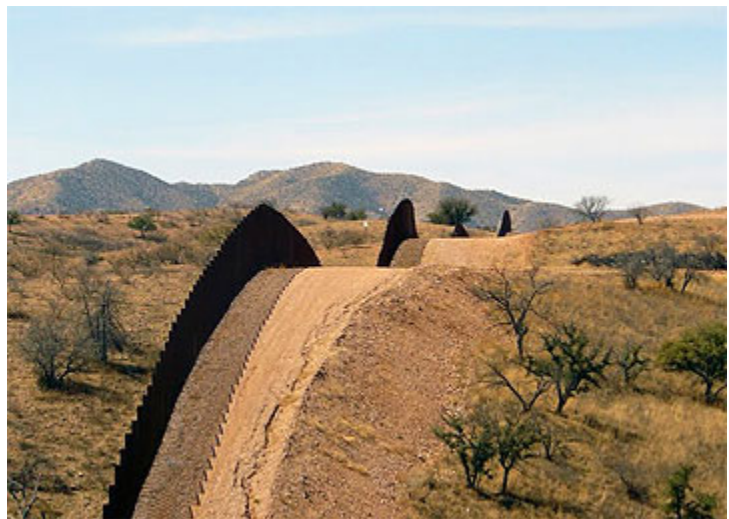
New border fence and access road west of Nogales, Arizona.
